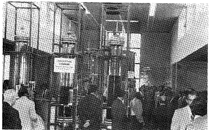
On Thursday, September 30, 1976, as part of the Convention Program the Philadelphia Water Department put into operation a UNIQUE PILOT PLANT — the first in any American city — to study advanced methods for removing trace organics from drinking water. Nearly 200 guests, including public officials, community leaders, and members of ASCE attended the brief ribbon cutting ceremony and a luncheon at the Torresdale Filtration Plant.
